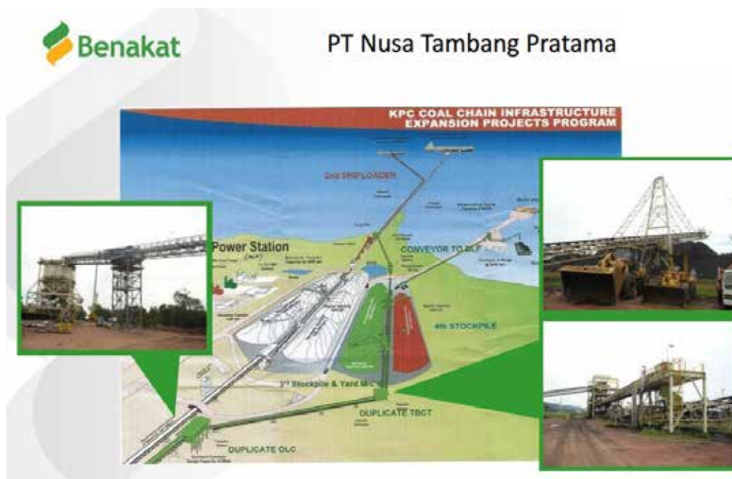
Duplicate OLC - Duplicate TBCT - Conveyor to BLF
